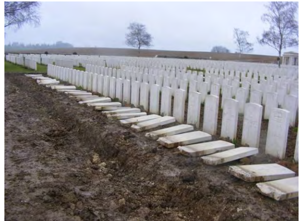
AIF Fliers – Work In Progress 2
