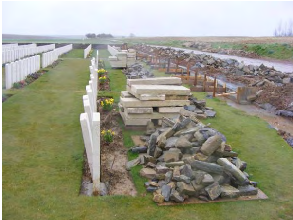
AIF Fliers – Work In Progress 1
