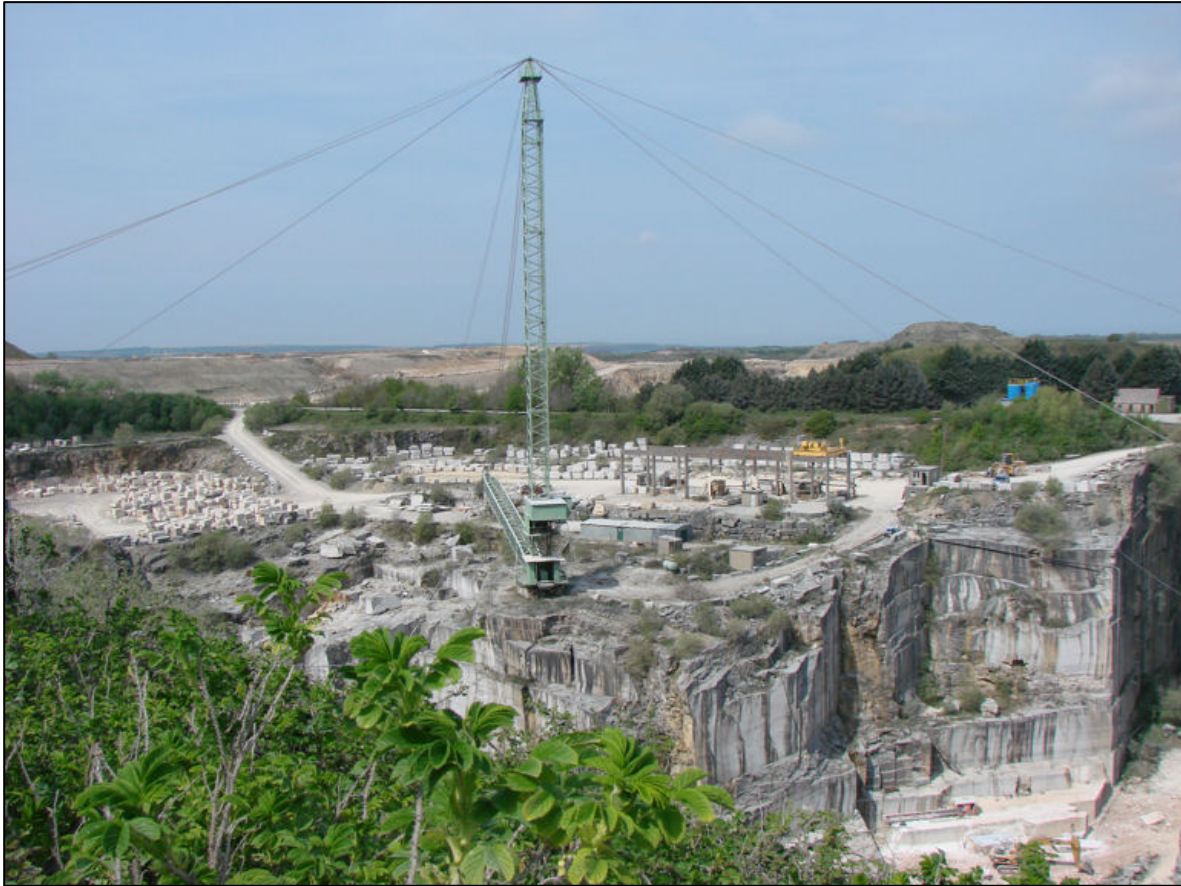
The Quarries at Marquise in 2007
