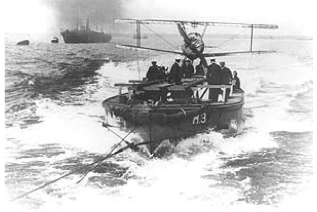
Lighter H3 with a Camel lashed down. The lighter was equipped with a cabin
