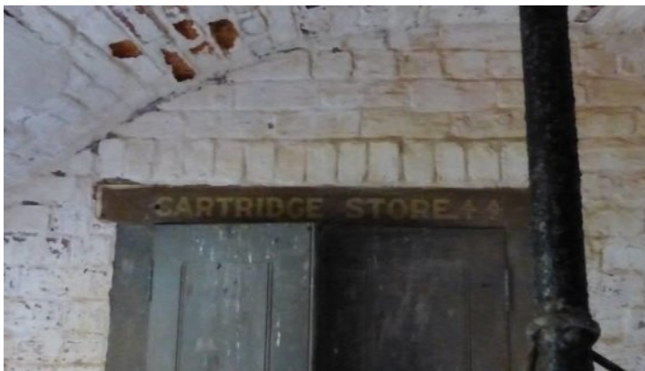
The Cartridge rooms of both Batteries (Above and Right)
